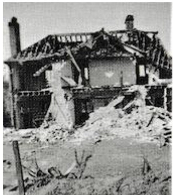
Whitecroft, Furze Grove showing V1 damage
