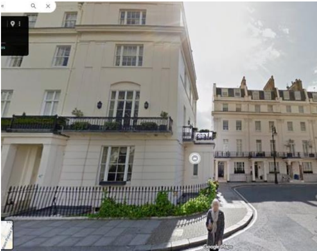
No 47 Chester Square is in the foreground left, No 45 is the 3rd house from the left in the background
